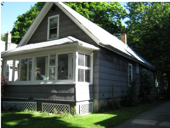
Roof & Siding Before
