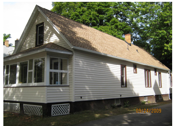
Roof & Siding After
